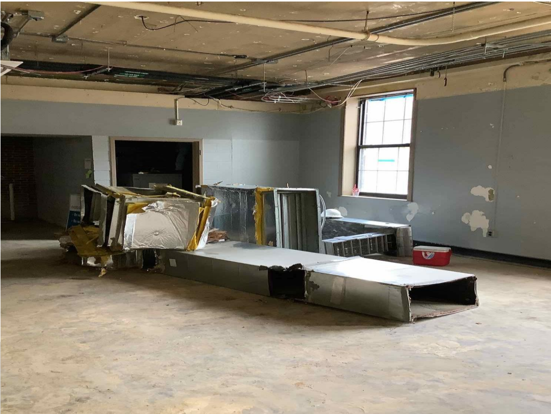
Mechanical demolition
